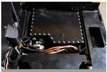
MINERAL INSULATED CABLES designed to meet needs of non-combustible, heat and water-resistant cable. Made of highly compressed mineral. The cables are sealed in a seamless copper tube, ensuring safety, making them liquid and gas tight. MI cabling provides flexibility and space saving.
